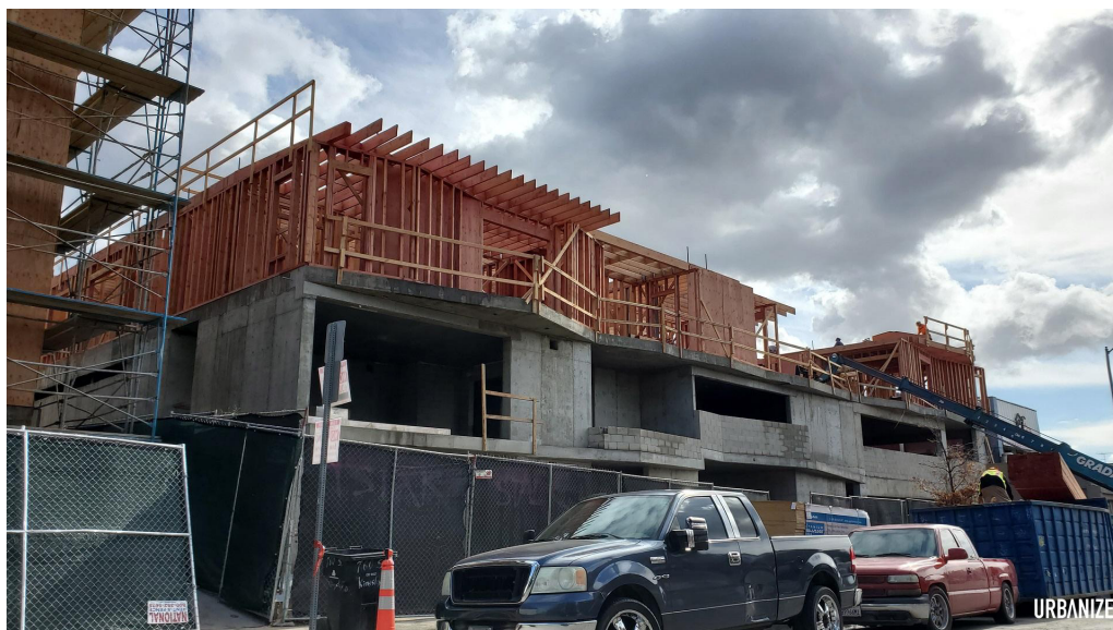
Construction at 750-762 S Kingsley Drive Urbanize LA
